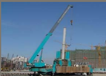
3. Pressing of bottom pile.
