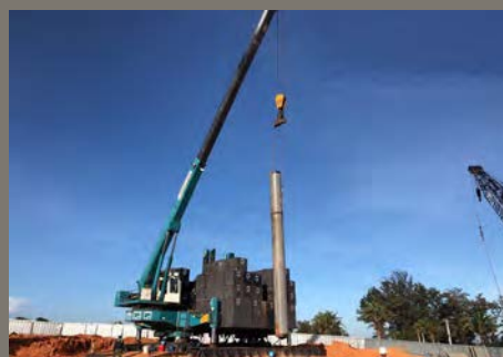
6. Pressing of top pile
