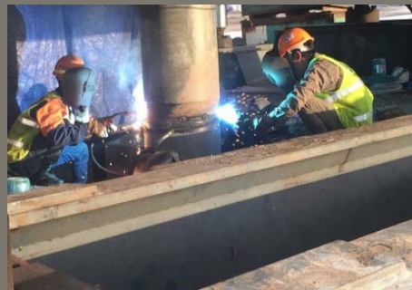
5. Welding of connection with steel plate.
