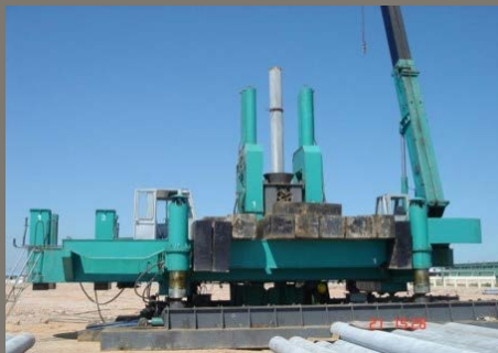
2. Setting of bottom pile and check verticality.
