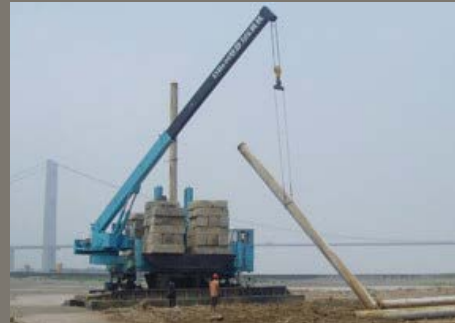
4. Setting of top pile and check verticality.
