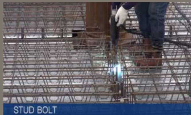
Deck anchoring
