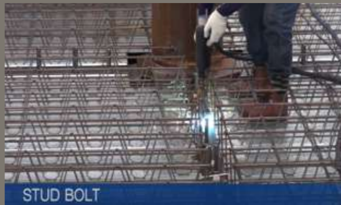
Deck anchoring
