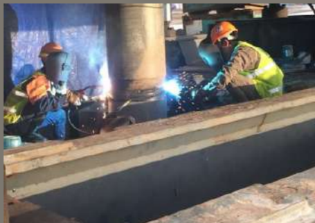
5. Welding of connection with steel plate. 5. Hàn nối cọc.
